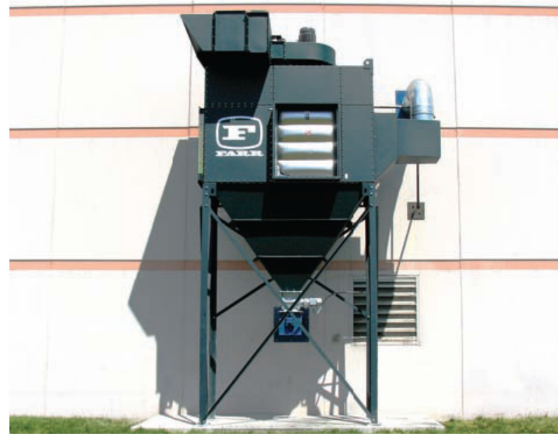
Cartridge dust collector with explosion venting to vent explosion away from building
